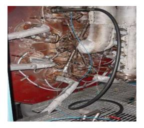
STF ENERGY is supporting customers in the worldwide plant and power generation market utilising our employee's significant technical experience in all aspects of engineering services. Our burner cleaning and flow testing services were originally developed for gas turbine burners but can be utilised to qualify any burner performance.
